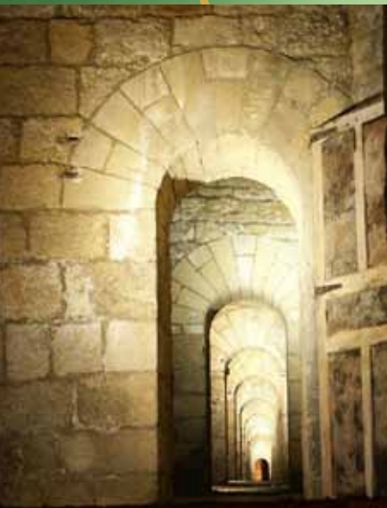
The underground galleries
